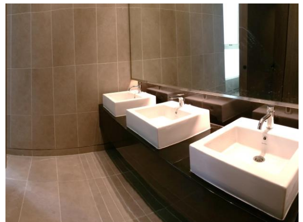
Newly Refurbished Toilets
